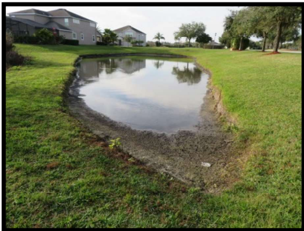
Figure 15 Pond 3 Shoreline Erosion
