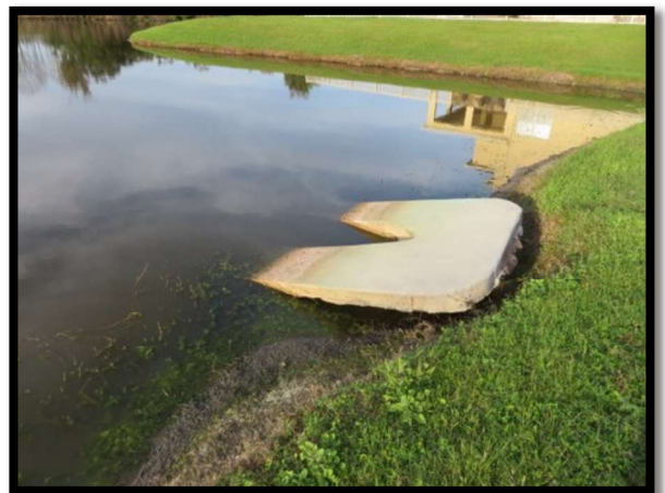
Figure 18 Pond 34 Shoreline Erosion
