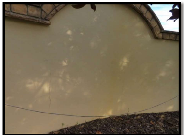
Figure 6 Stucco Cracks and Faded Paint
